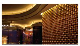
2800°K LEDs, 2" on center spacing were mounted at a 45° angle in individual mounting brackets for each LED module to facilitate the corner turns and ensure consistent beam angle of the light.
