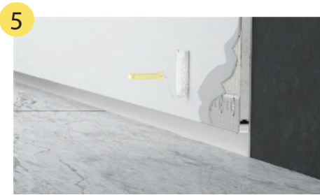
5 After drying - finish with paint coat
