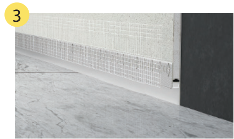
3 Stick mesh-tape on extrusion and drywall evenly divided on both surfaces
